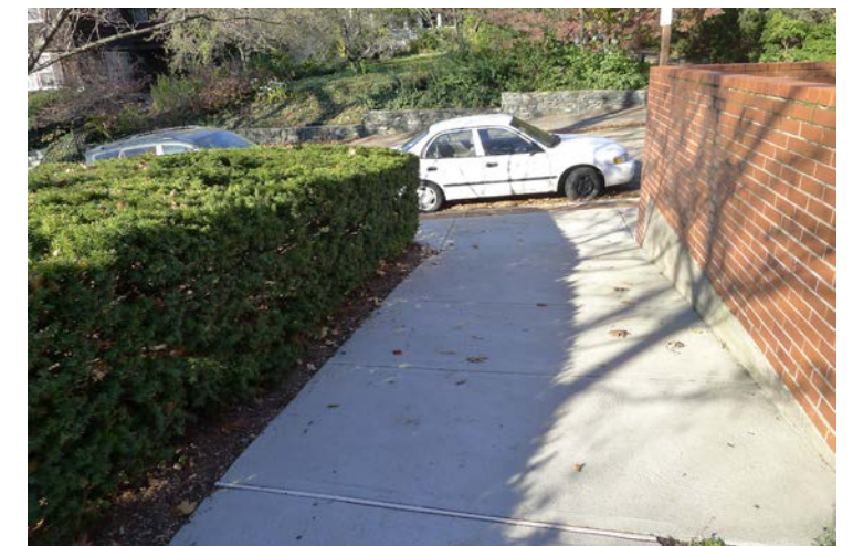
N Slopes are too steep.
