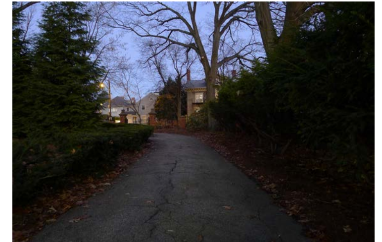
F Insufficient lighting along pathway.
