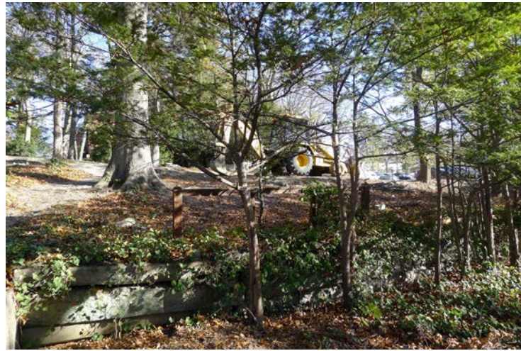
A Terrace disconnected from site and in poor condition
