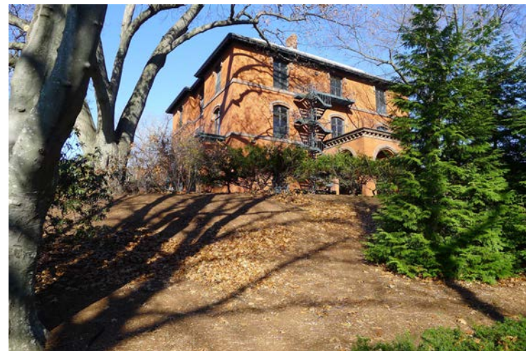
B Bare soil creates erosion issues.
