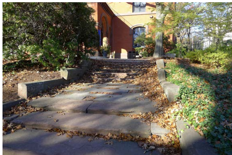
J Brownstone stairs are deteriorating
