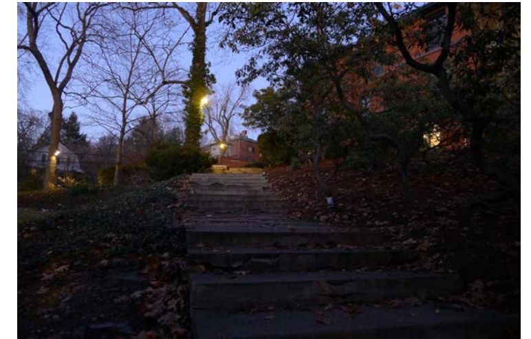
A Lighting in trees creates maintenance and safety problem. Too high.
