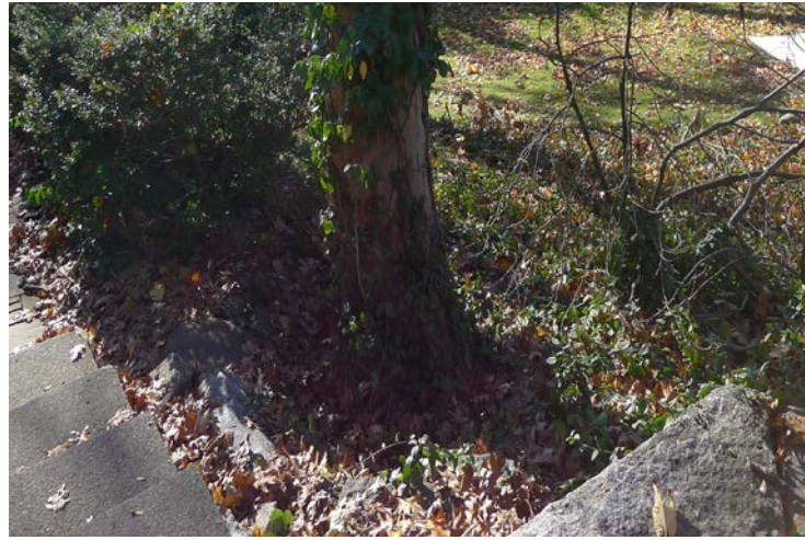
A Erosion against stair edge. Euonymus damaging trees.
