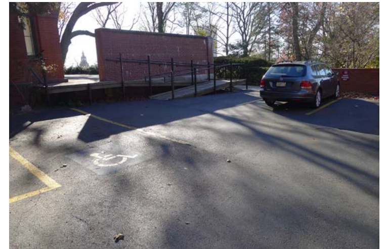
L HC parking needs to be reconfigured.
