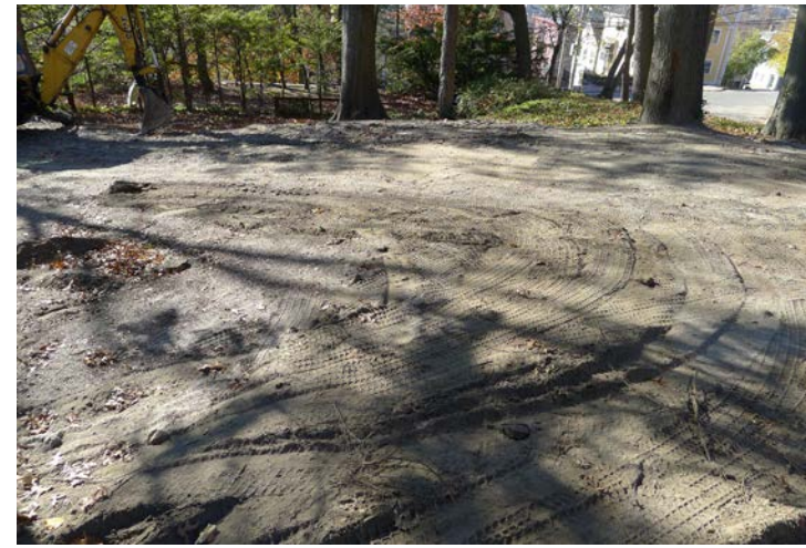
C Road bisects and cuts off site.
