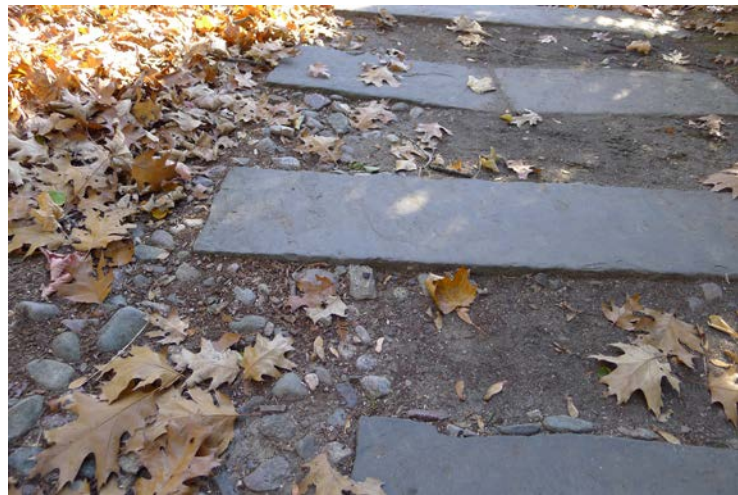
E Gravel is eroding around granite
